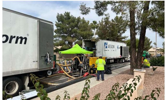
Dibble and Dibble CM provided onsite construction inspectors
