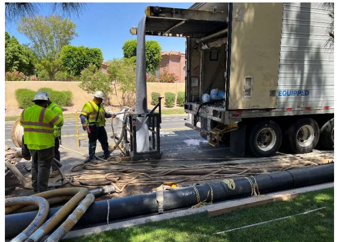
Installation of the CIPP liner
