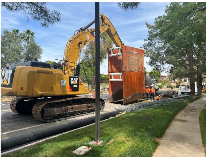
Construction along Jacaranda Parkway
