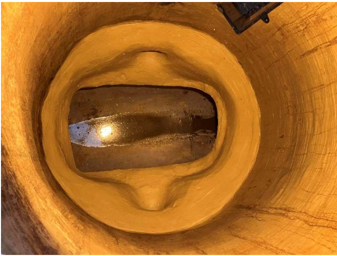
Manhole rehabilitation work was completed on 13 manholes
